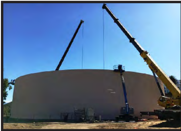
Pictured HP Reservoir Rehabilitation Project Top: New Roof Installation; Bottom: New Interior Staircase
