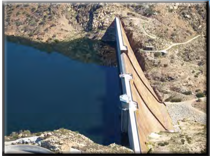
Pictured: San Vicente Dam and Reservoir Photo credit: San Diego County Water Authority
