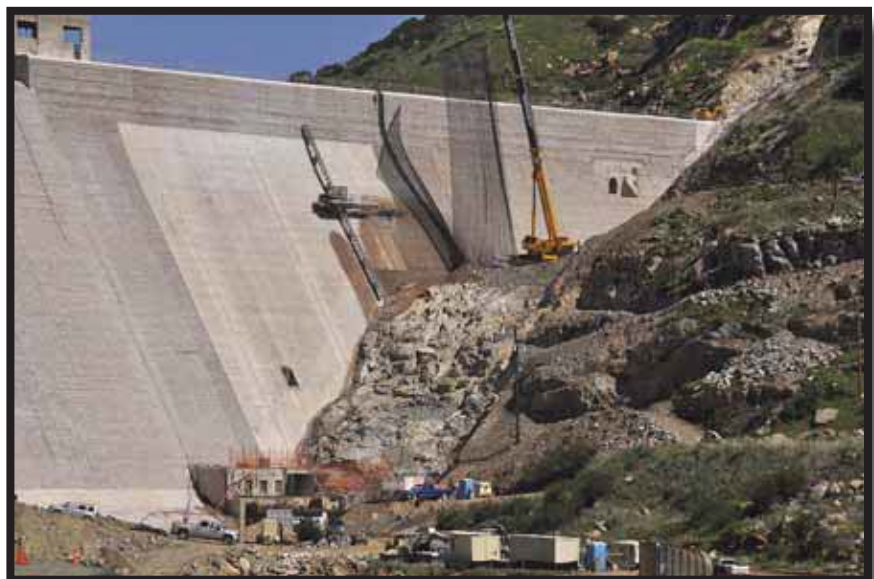
San Vicente Dam under construction
