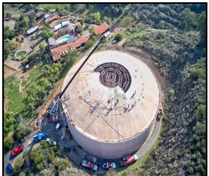
Pictured: Aerial view of HB Reservoir Project in progress
