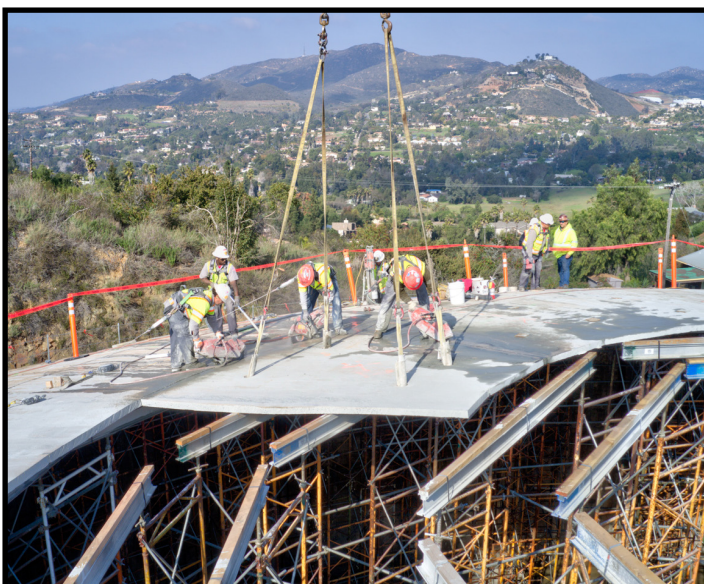
Pictured: HB Reservoir roof demolition in progress
