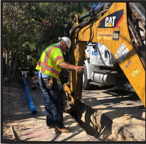
Pictured: Mainline Replacement on Montgomery Drive
