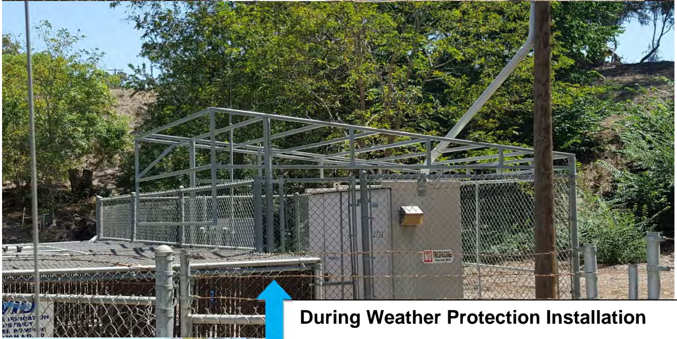
Before Weather Protection
