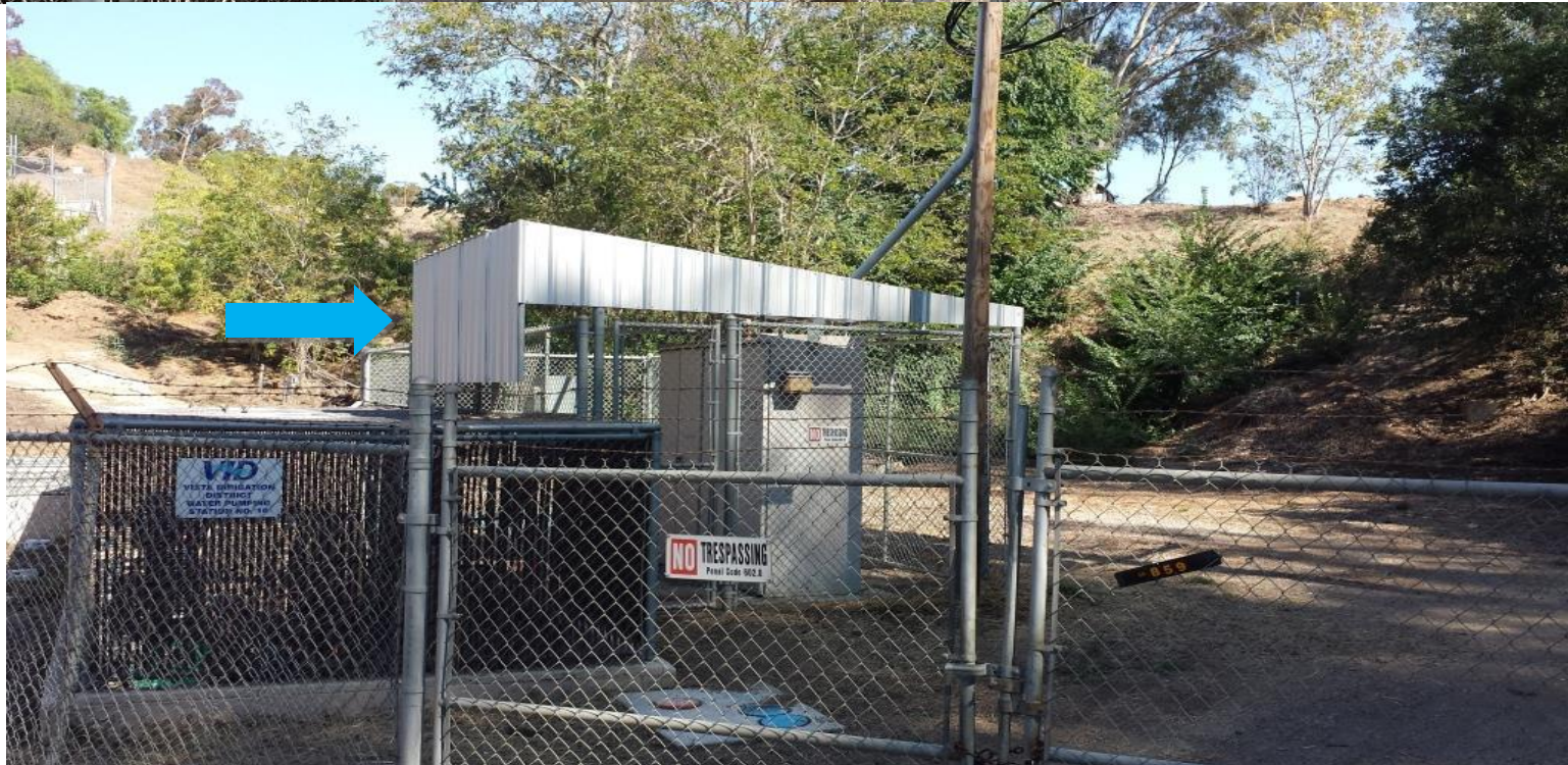
This photo shows the newly installed cover.
