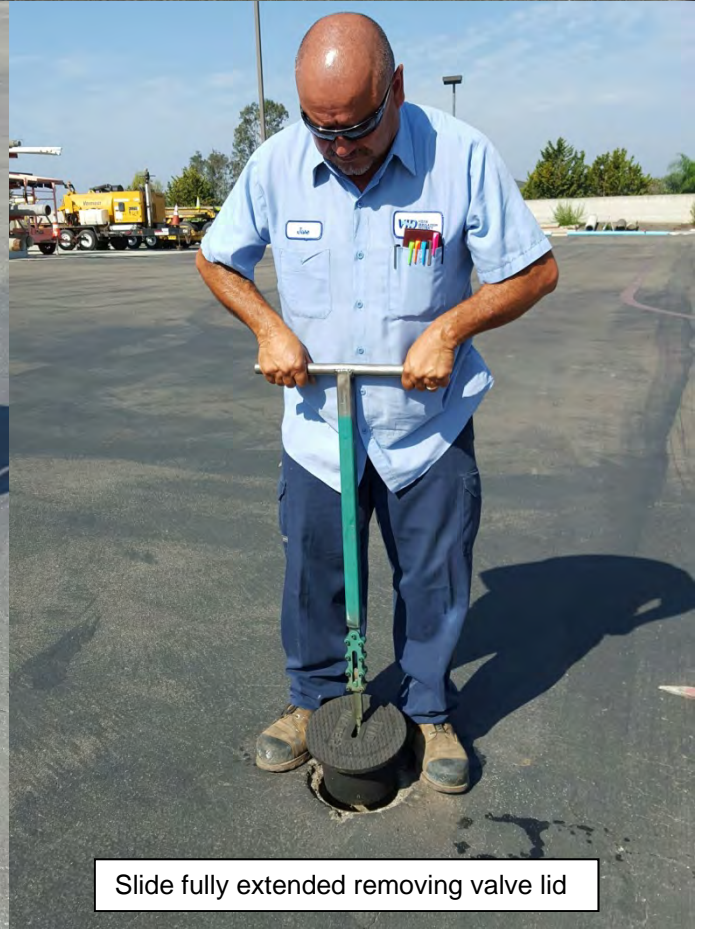
Traditional valve lid removal method – non slotted
