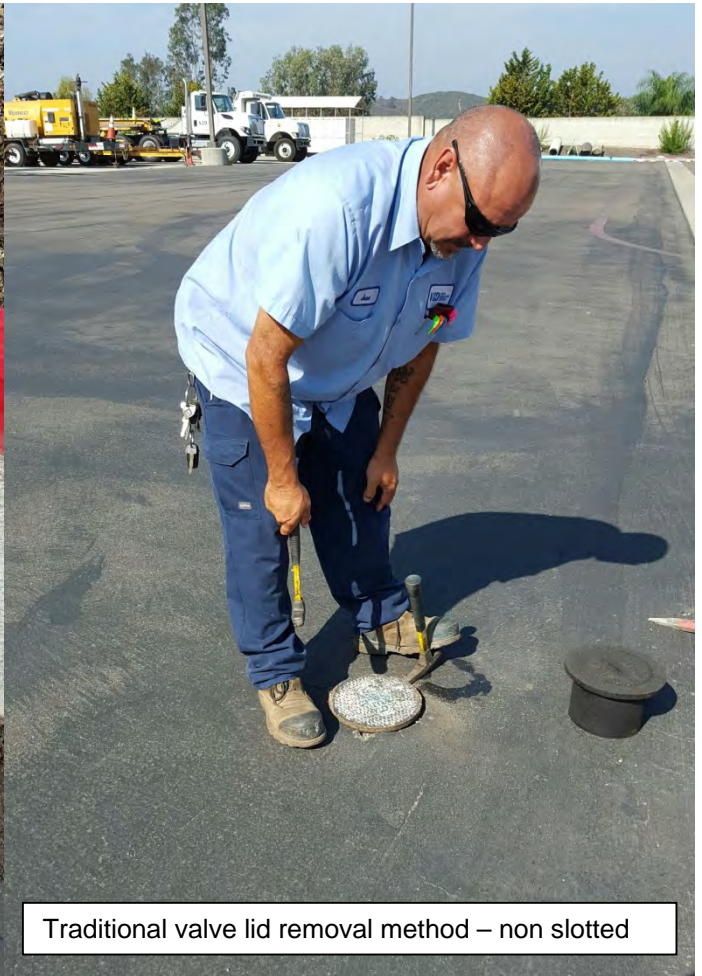
Rock pick hammer, final and initial lifting tool design
