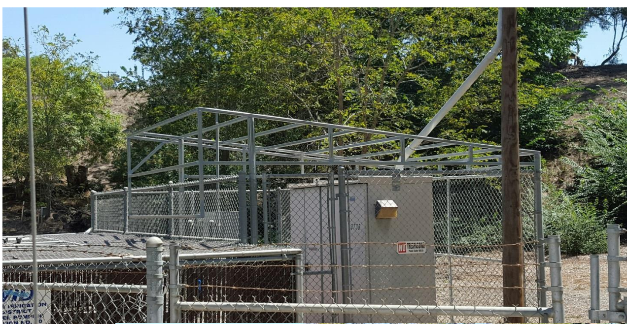
This photo shows the framework for the new cover.
