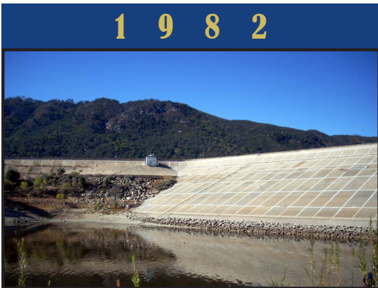
Henshaw Dam is re-engineered for seismic reasons, reducing the lake's capacity from 200,000 acre feet to 50,000 acre feet.
