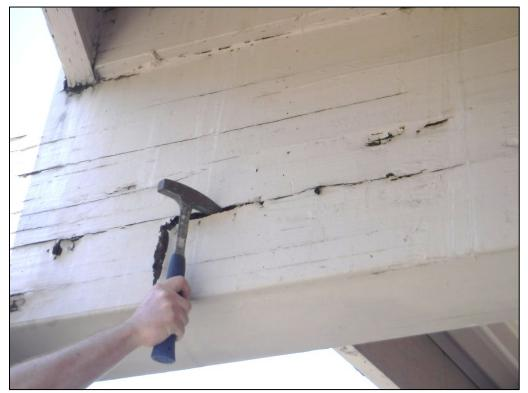
Photo 16 – Valley beam 29 where significant pockets of dry rot were found, greater than 3" deep in some areas.
