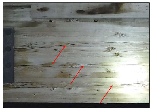
Photo 13 - Close up of the checks seen in Photo 12 pointed out by the red arrows at valley glulam beam 21 between purlins L and K.
