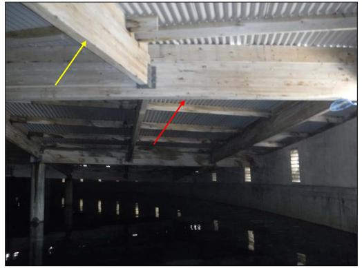
Photo 9 - Typical ridge glulam beam 11 (red arrow) between purlin L (yellow arrow) and cmu wall.
