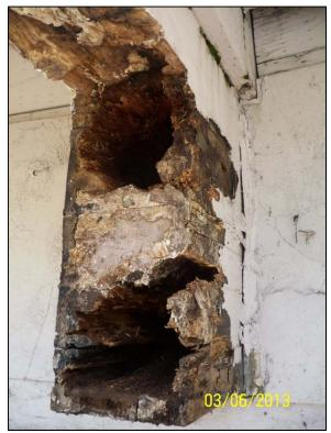
Photo 21 - Valley glulam beam 13 during maintenance repair in 2013, provided by VID staff.
