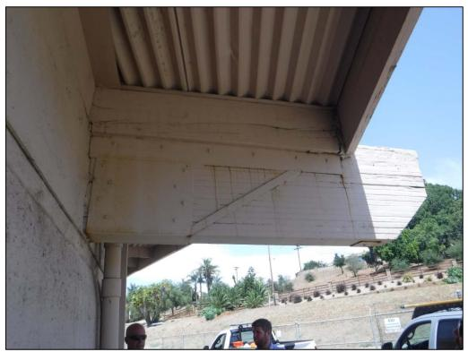
Photo 20 – Repaired portion of valley glulam beam 13.
