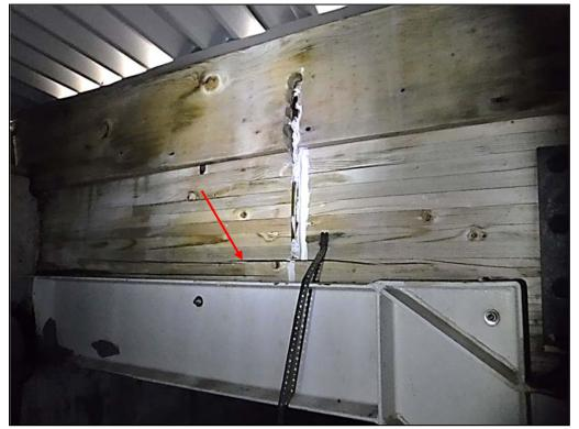
Photo 19 – Split at valley beam 13 between cmu wall and purlin L.
