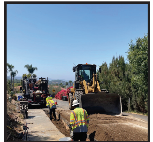
Pictured: Mainline Replacement on Vista Grande
