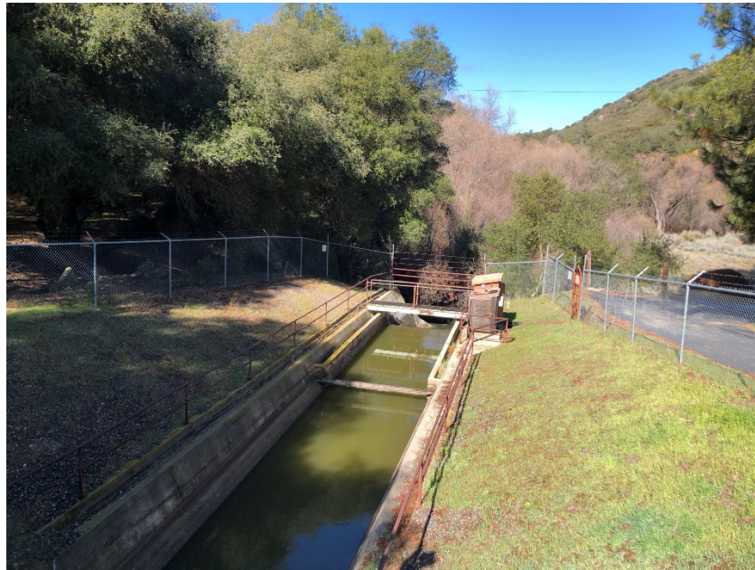
Figure 4. Henshaw Dam outlet channel to the San Luis Rey River.
