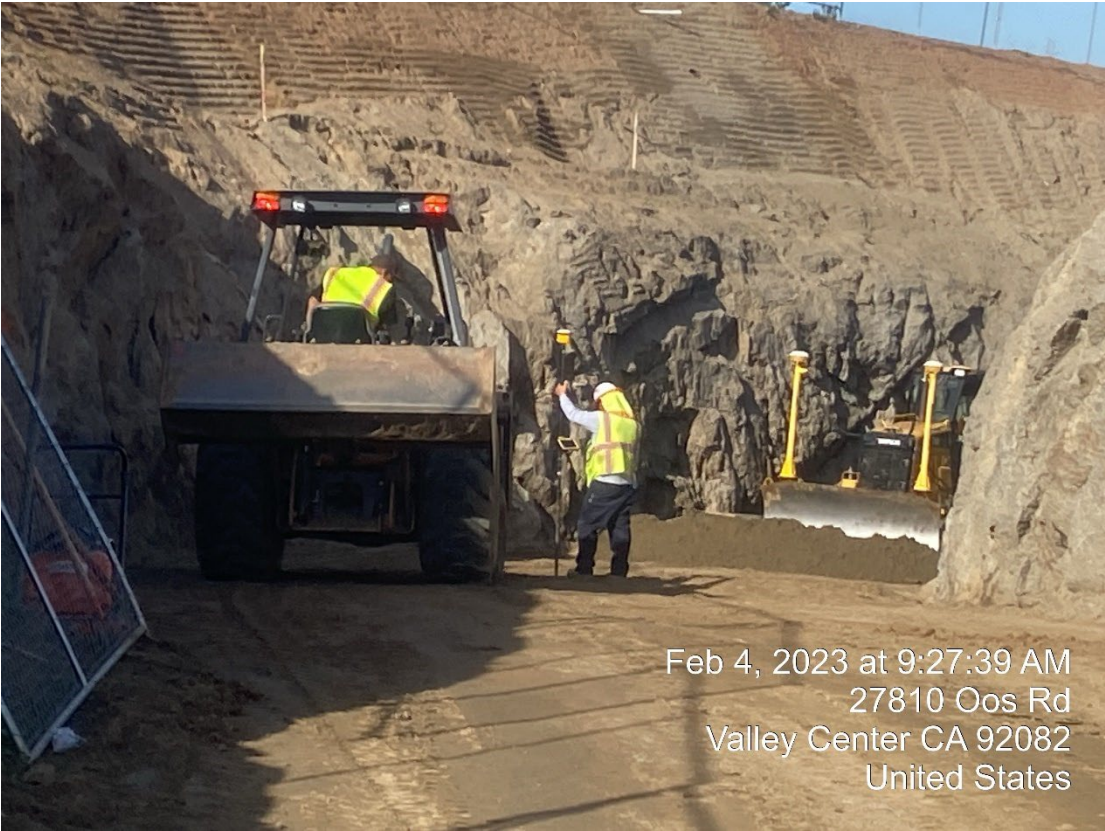
Final grading of access tunnel
