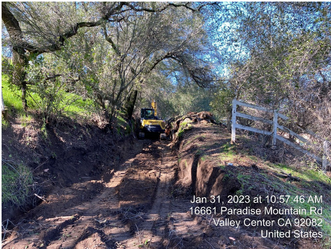
Remaining canal demolition
