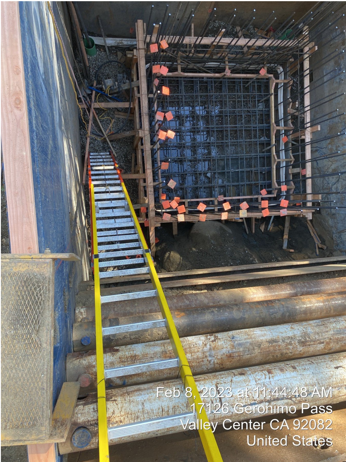
The rebars and forms for the drop structure base
