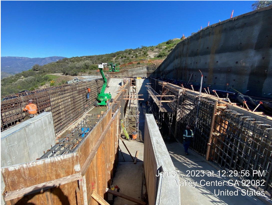
Final rebars and forms inspection prior to next day's pour
