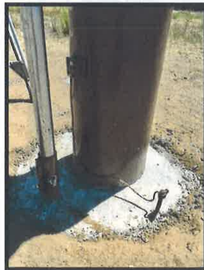
A close-up of the grounding rod, which prevents equipment damage from lightning strikes.
