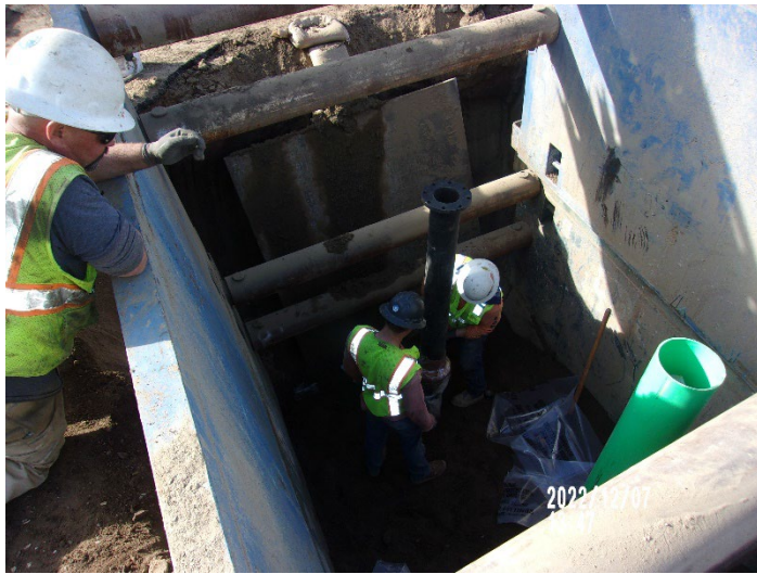
Installing the blowoff valve for the Pump-out structure
