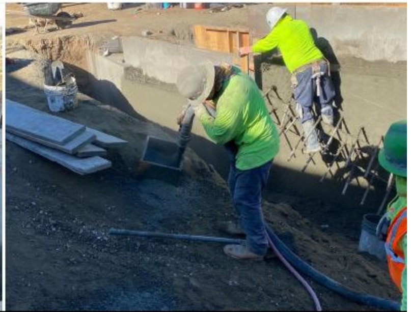
Shotcrete for the inlet/outlet wall structure for the desilting basin took place on Saturday 12/10
