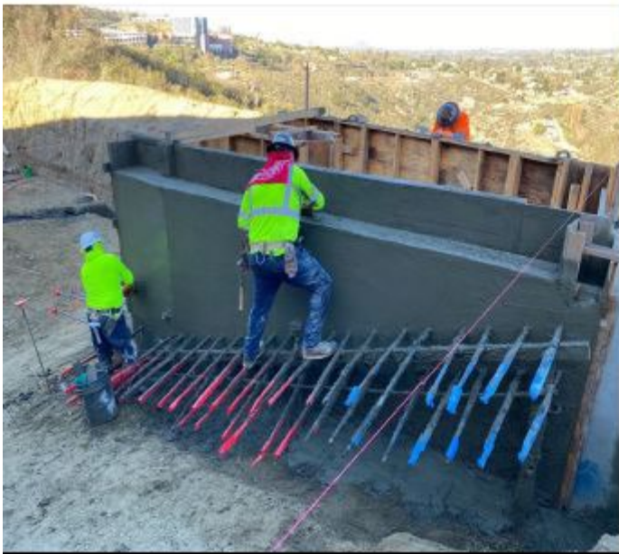
Shotcrete for the inlet/outlet wall structure for the desilting basin took place on Saturday 12/10
