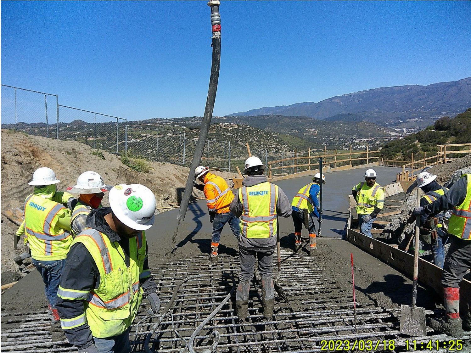
The concrete pour for the first half of the access runnel
