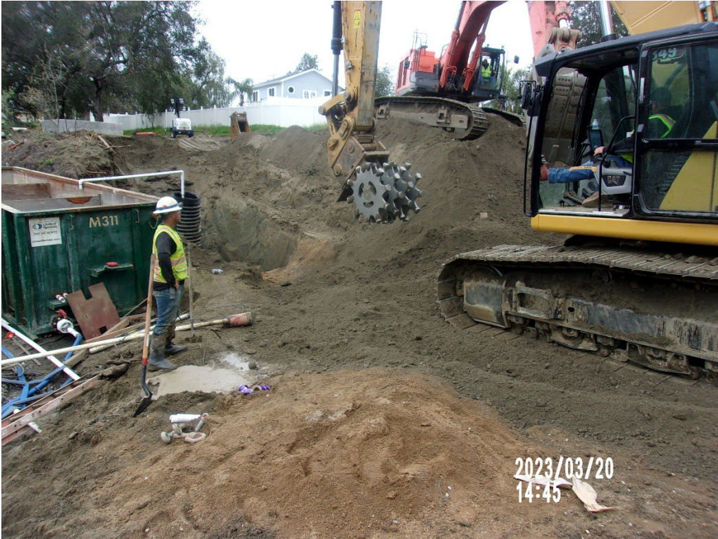
Last pipe installed as of Monday 3/20
