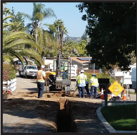
Pictured: Mainline Replacement on Rosario in Vista
