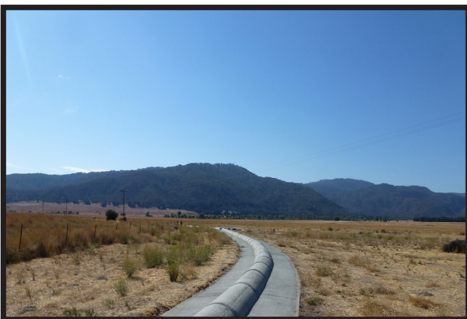
Local Water Source: 36" Reinforced Concrete Pipe conveys water from the District well field to Lake Henshaw Photo credit: S. Thorpe
