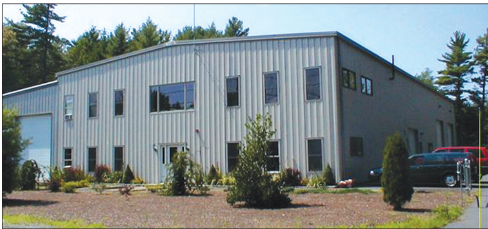
The Warren Companies' facility, located in Middleboro Mass.
