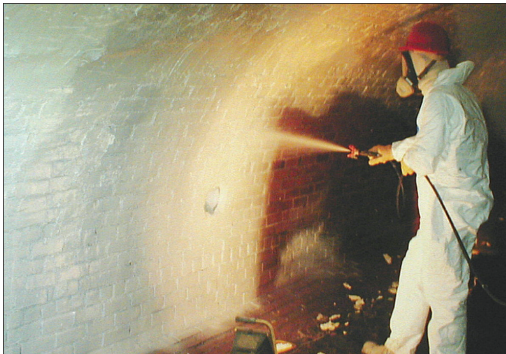
Boston tunnel spray application.
