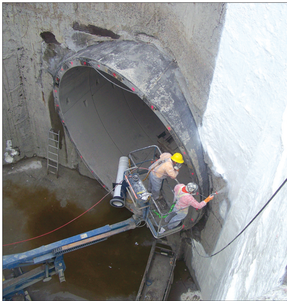
Repairing a 100-year-old brick tunnel in Boston.
