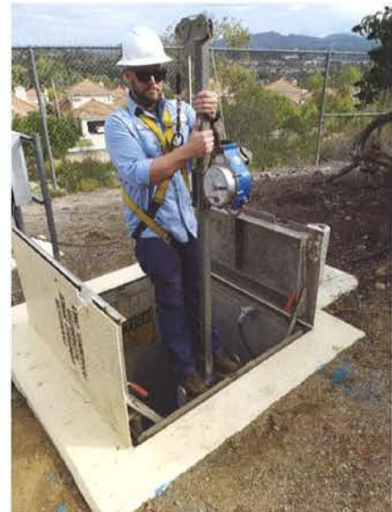
Vista Irrigation District – The district cut a small opening in the vault lid directly above the fall protection receiver and installed a hinged cover to secure the opening and the receiver when not in use. The design allows the davit arm to be attached to the receiver and the employee to be tied off prior to the vault lid being opened.
