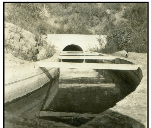
Flume exiting Big Tunnel, circa 1930's - 40's
