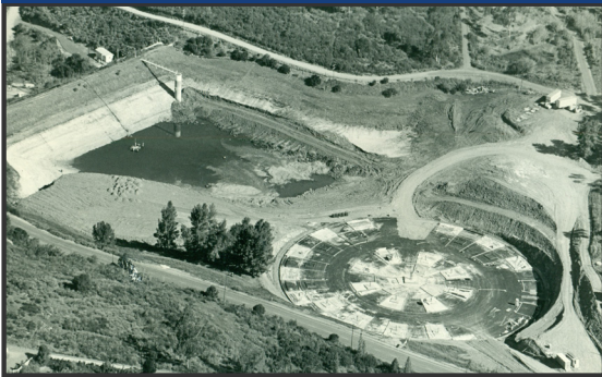
Pechstein Lake is replaced by the covered Pechstein Reservoir.
