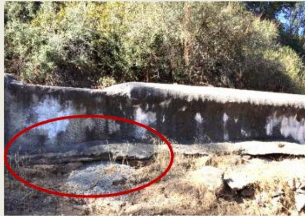
Not suitable for reuse. Left : Roof separation, Borden Bench; Right : Erosion under Daley Bench
