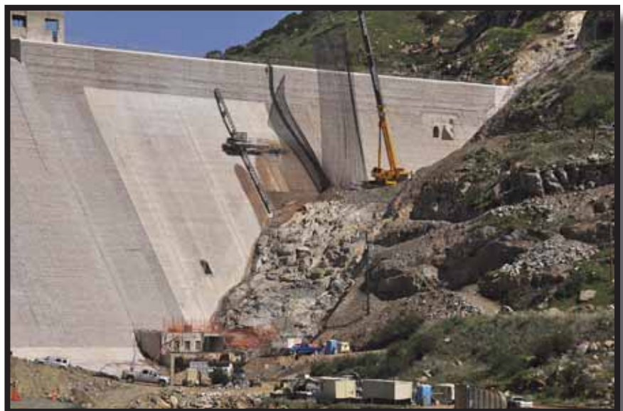
San Vicente Dam under construction
