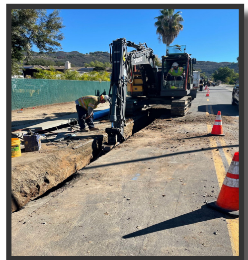
Mainline Replacement on San Clemente Ave
