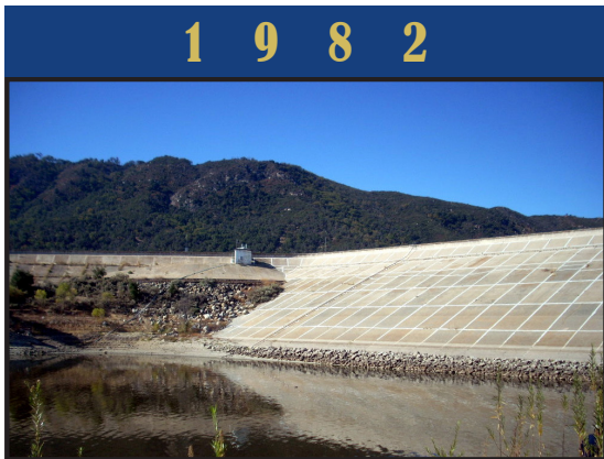
Henshaw Dam is re-engineered for seismic reasons, reducing the lake's capacity from 200,000 acre feet to 50,000 acre feet.
